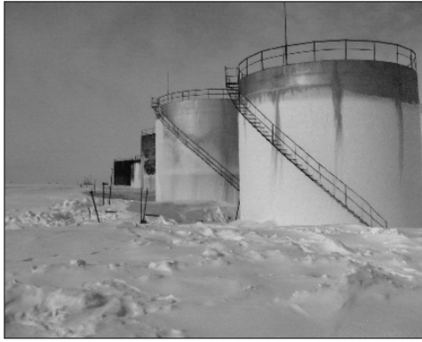
(← Fig. 6.7) The onshore tank farm
