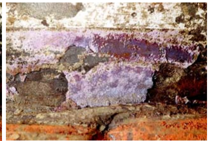
Fig. 23. after removal off the glossy material with acetone, Nov. 1, 2000
