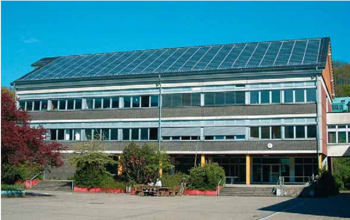
Figure 1: The Aggertal-Gymnasium secondary school, Engelskirchen, is one of the solar schools that save money and energy (Source: Wuppertal Institut)
