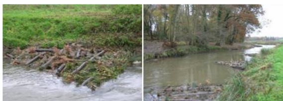
Fig. 1 Narrowing of the channel using wooden wing deflectors (from Hammond et al. 2009).
