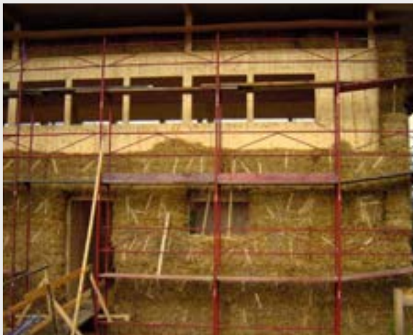
Demonstration building S-House (Source: GrAT)
