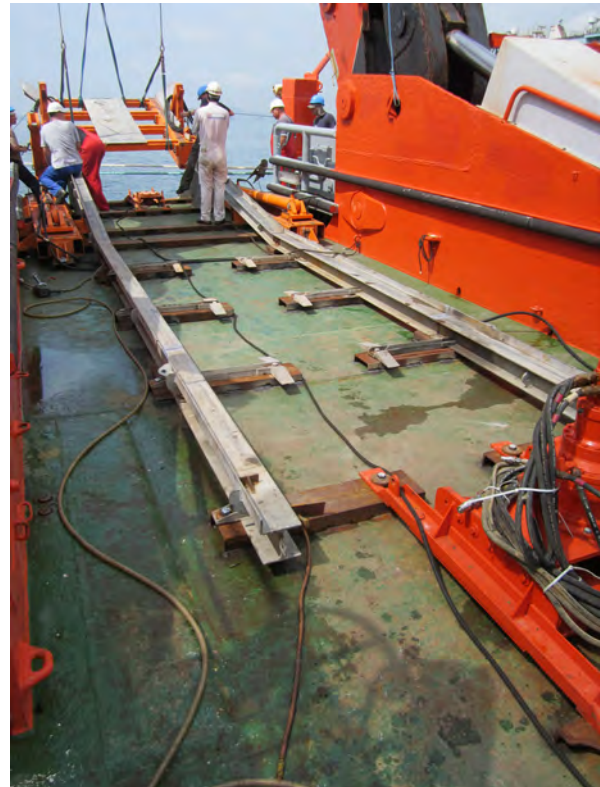
Fig. 3.2:. Basal frame for the MeBo Launch and Recovery System beneath the ship's A-frame.
