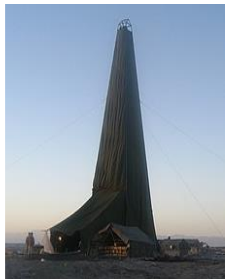
Fig.6: View on the veiled drilling rig in the Jianshan anticline during winter times.
