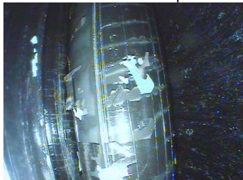
spallations at cladding at 400 mm
