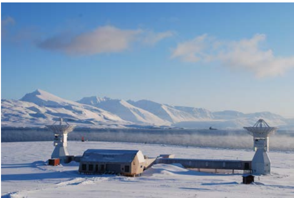
Figure 5. The twin VLBI antennas of the new observatory in Ny Ålesund, Svalbard (Photo: Norwegian Mapping Authority)
