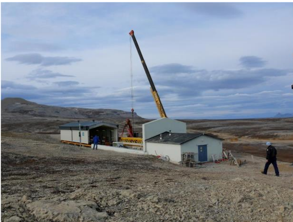
Figur 4 - Installation of the U4 launcher in Ny-Ålesund in 2008
