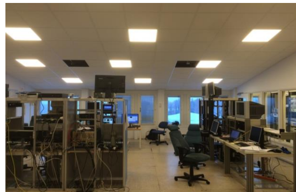
Figure 6. TMC; A new ceiling with dimmable LED-lights was installed.
