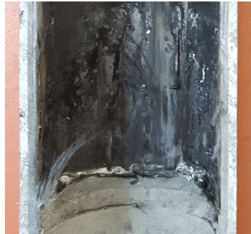
Figure 4: Deterioration of casing after test 3
