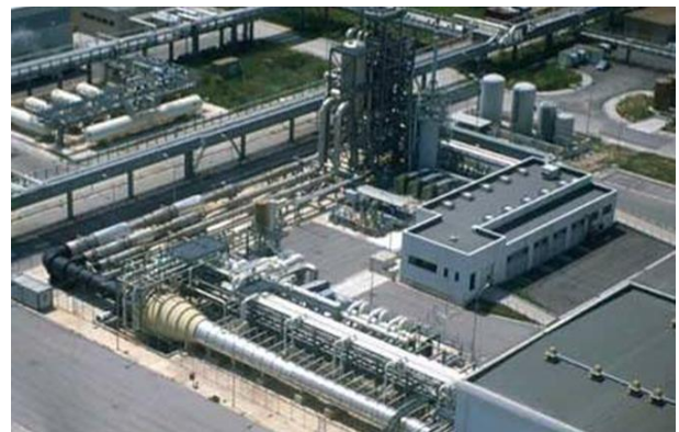
Figure 15. SCIROCCO facility aerial view
