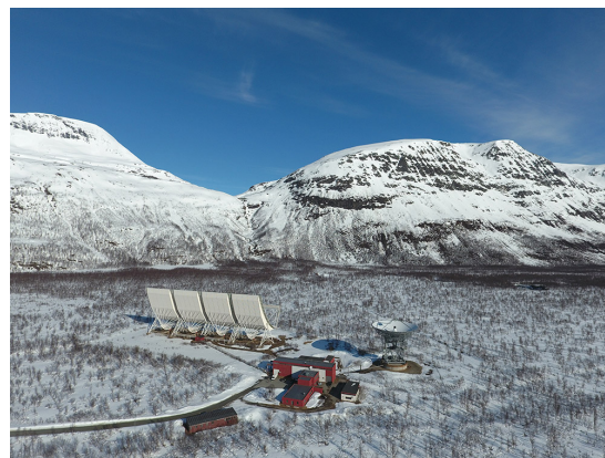
Figure 3. The main EISCAT mainland site at Ramfjordmoen near Tromsø in Norway. From left to right the VHF 120×40 m antenna, the main building, and the 32 m UHF dish can be seen. The Heating and ionosonde antenna arrays are outside this picture.
