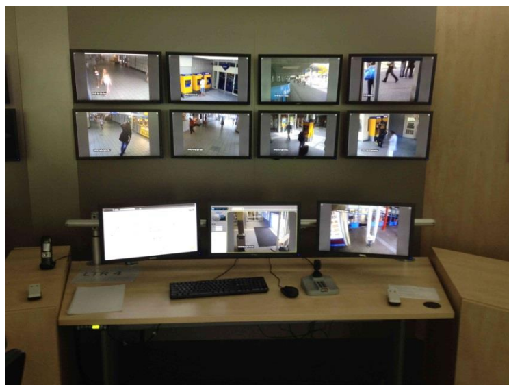
Figure 7. Railway station surveillance centre. The top eight images display separate locations in the station. Each image represents a separate scene.
