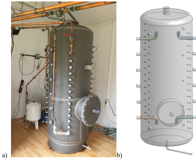
Fig. 2. Water tank for thermal energy storage (a) and its geometrical model (b)
