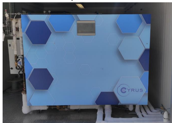
Fig. 5. Metal Hydride Compressor
