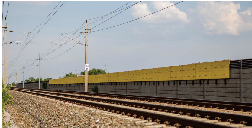
Figure 1: Modified noise barrier. Shown is the upper panel configuration.
