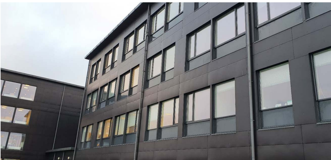
Picture 3 Continuous measurement at facade of office building
